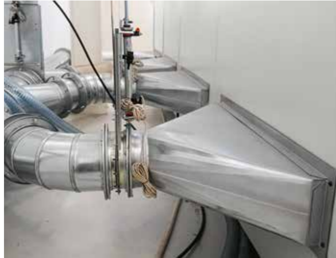
Dust extraction system for effective air recirculation and combating dust inside the work area
